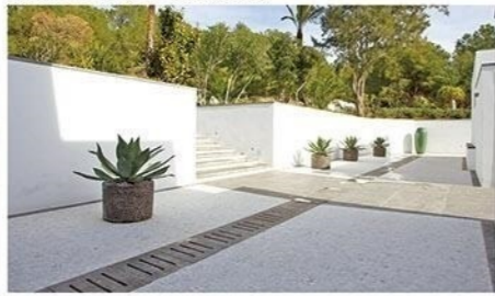
PAVING & DITCH STONES
