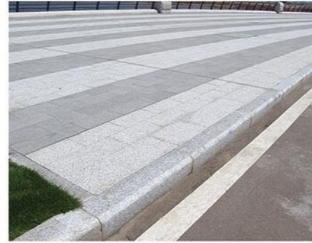
G654 & 603 PAVERS & CURBS PROJECT
