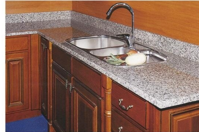
KITCHEN COUNTER TOPS / SESAME WHITE GRANITE
